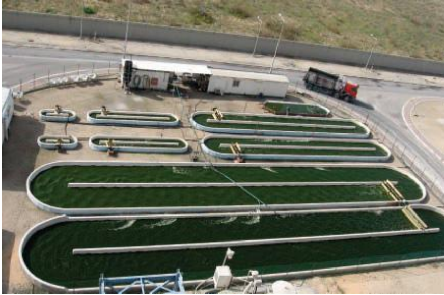
Figure 22: Open-pond Test Facility at Ashkelon ( Seambiotic )
